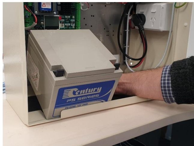
Figure 2: Installing the first battery
